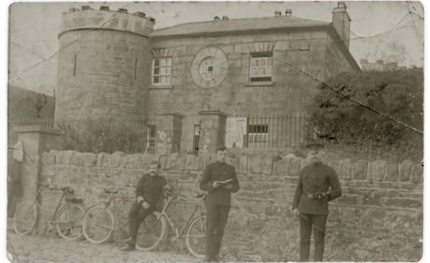
● Ballinamuck R.I.C. Barracks, County Longford (BMH/P2/001).
